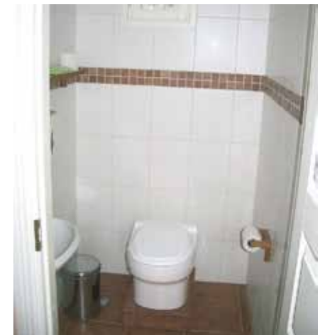
The toilet facilities are located at the upstairs and the composting chamber downstairs.
