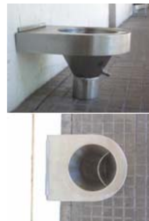
Fig. 4 – Urine Diverting Toilet
