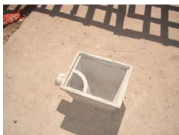
Fig. 6 – Solid Matter and Grease Intercepting Chamber
