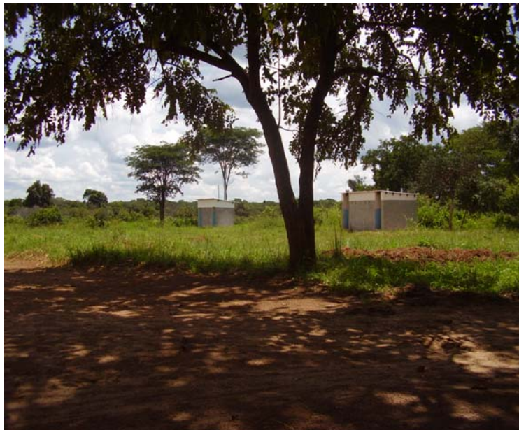
Figure 3. Covered pit latrines at Chisapa community
